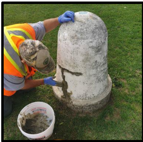
Figure 10 – Daniel Laviolette repairs a bell-shaped monument (NY/ON)
