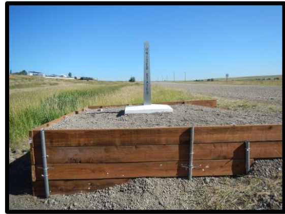
Figure 16 – finished retaining wall around base (MT/AB)
