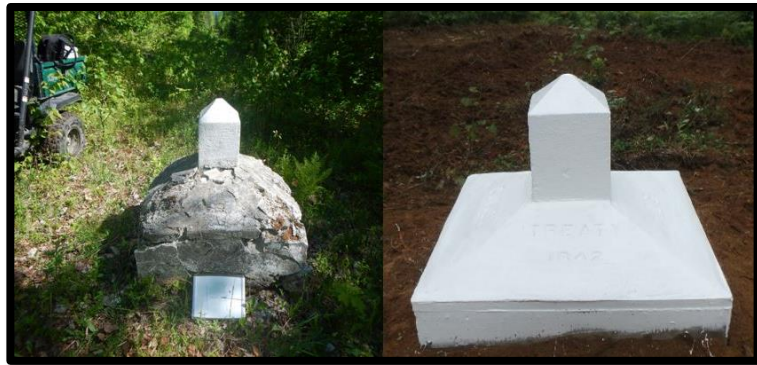
Figure 2- (Left) Mon 1B as recovered and (Right) Mon 1B after renewal (ME/NB)
