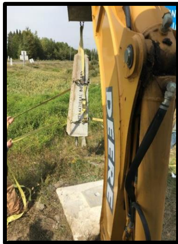
Figure 3- Setting the obelisk in place with a backhoe (ME/NB)
