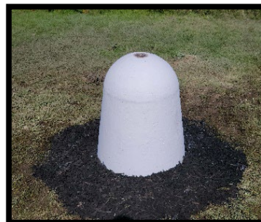
Figure 11: Reference Monument 32-41 as renewed in its original position (ON/NY)
